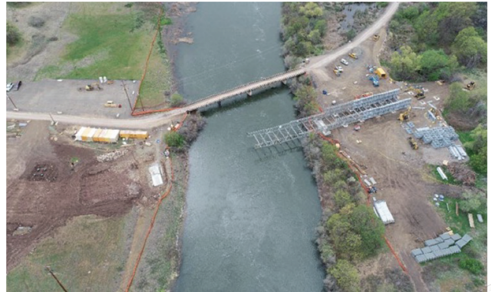
Daggett Bridge Work
