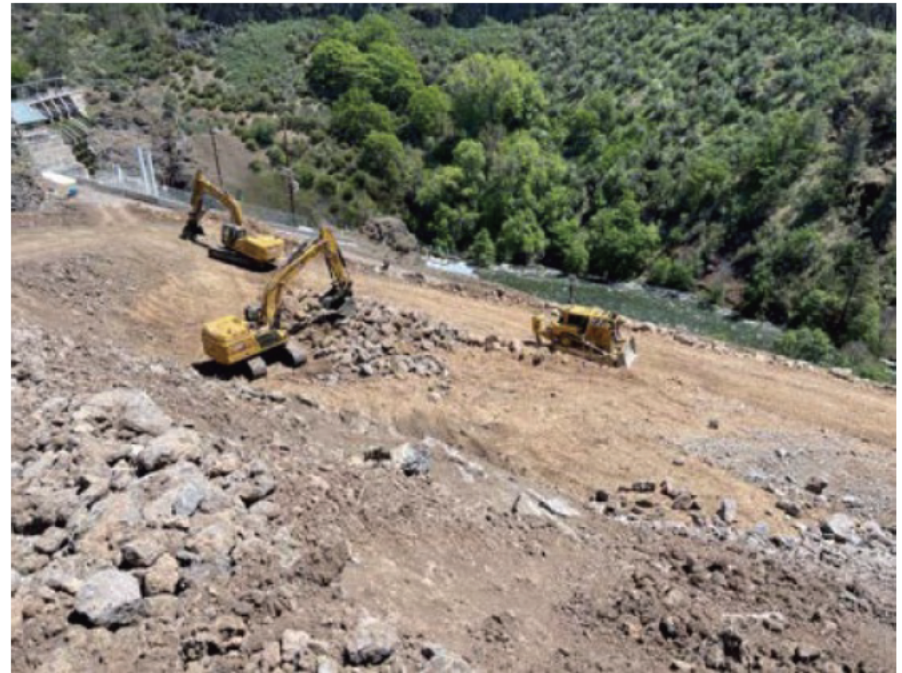
Copco No. 1 Access Road Work
