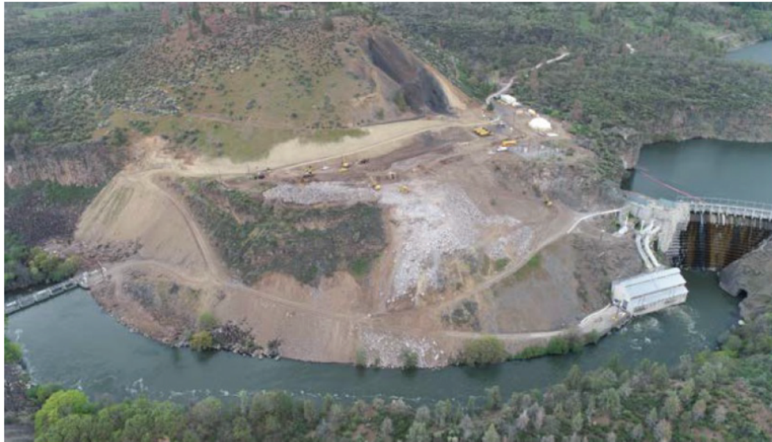
Copco No. 1 and No. 2 Access Work
