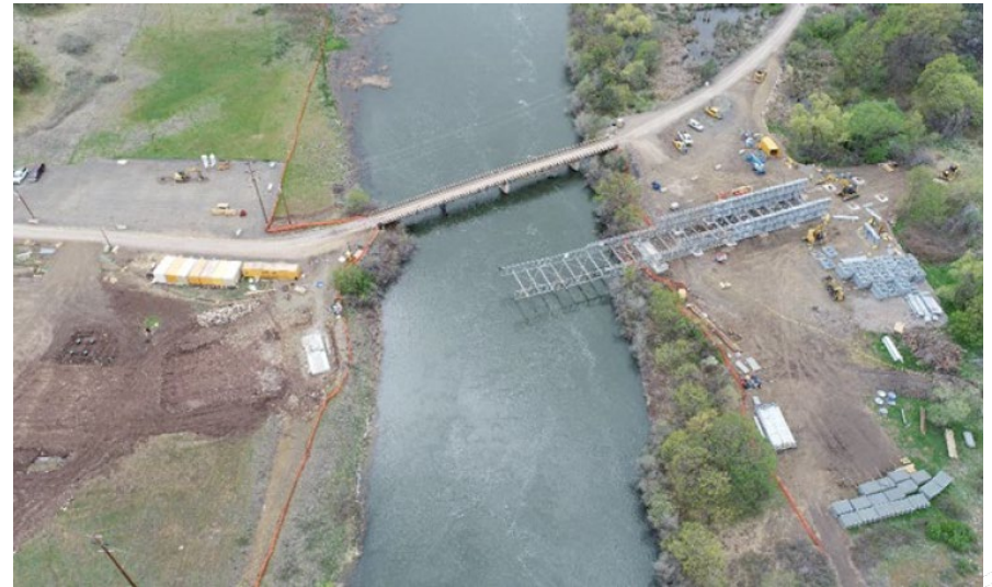
Daggett Bridge Work
