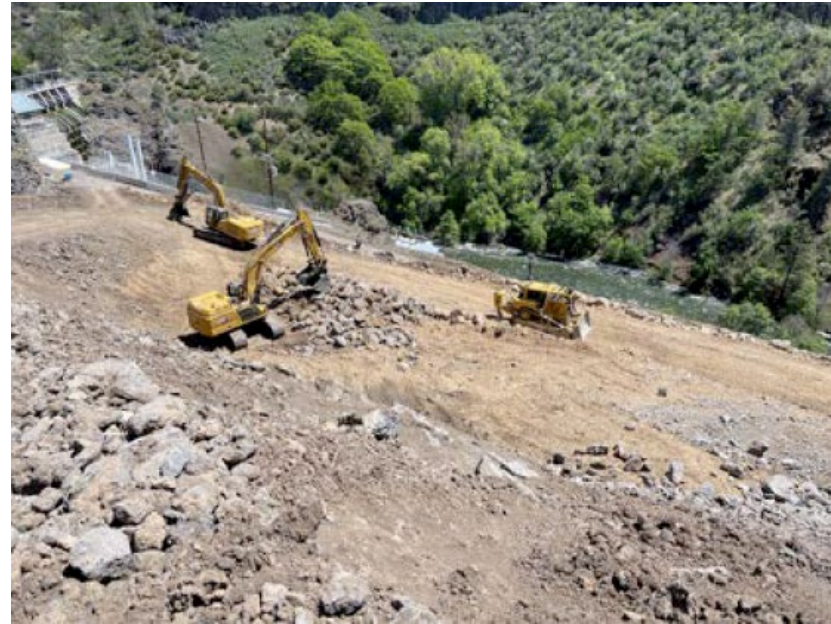
Copco No. 1 Access Road Work
