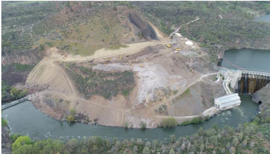
Copco No. 1 and No. 2 Access Work
