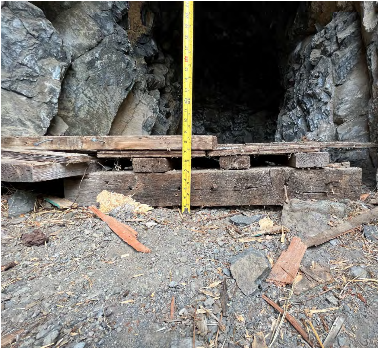
Photograph 7: Plywood Floor with Support Beams
