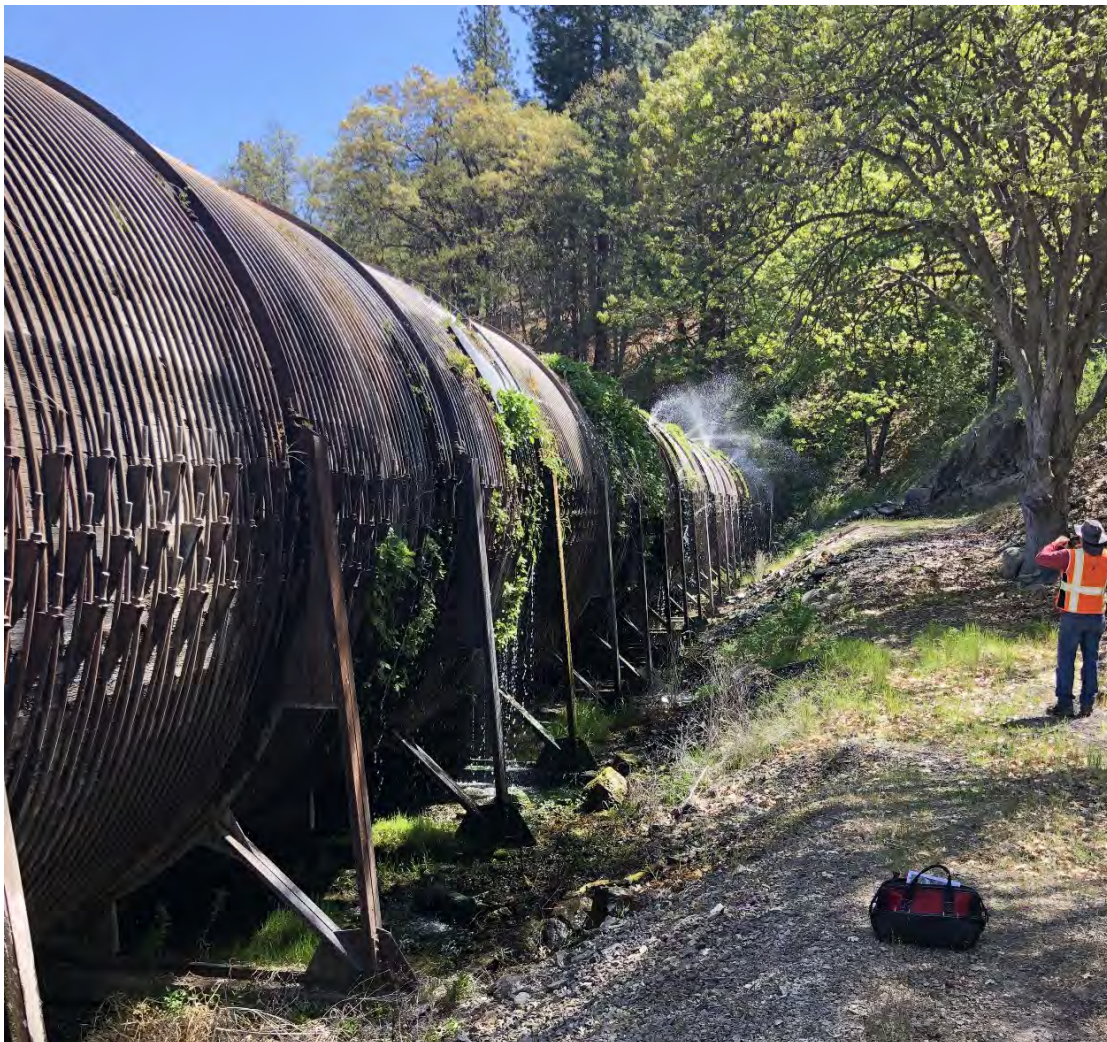
Photograph 6-1. Copco No. 2 Wood-Stave Penstock (Jacobs 2022a)
