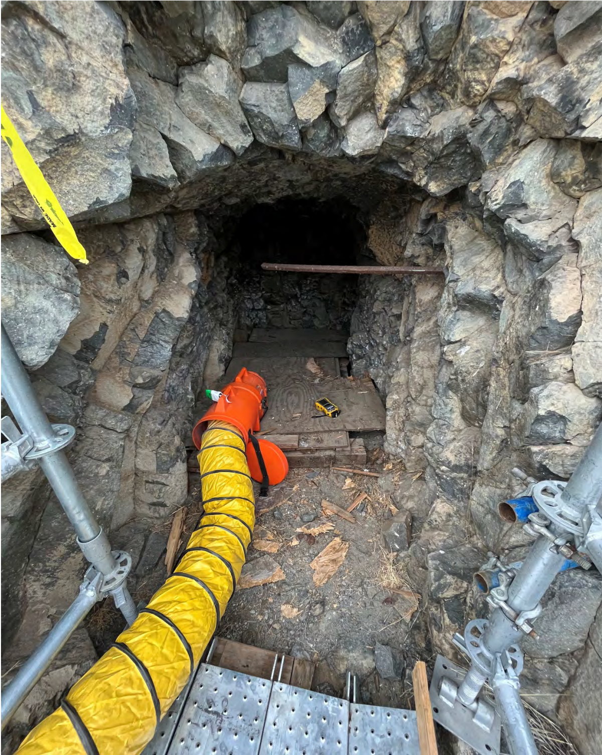
Photograph 2: Cave Venting and Air Monitoring, View 2
