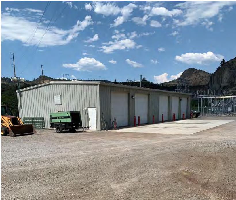
Photograph 9-1. Existing Maintenance Building (Jacobs 2021a)
