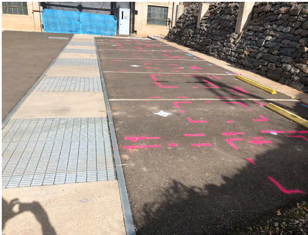
Photograph 8-1. Location of Four Boreholes (white paint) and Underground Anomalies (pink paint) at the Former Transformers (Jacobs 2022a)
