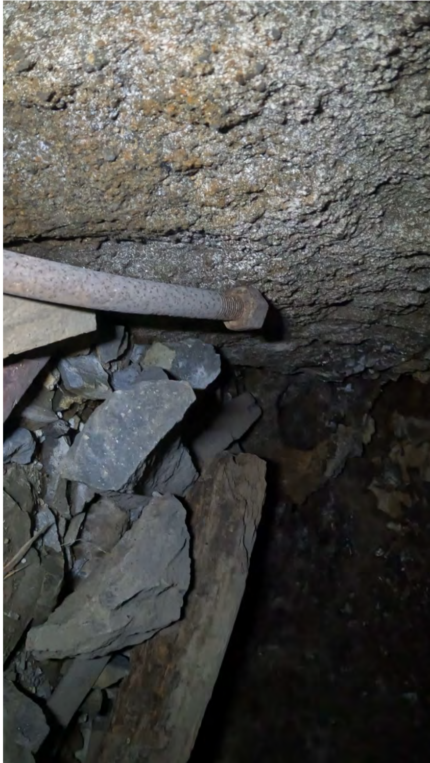
Photograph 9: Shaft Debris View 1
