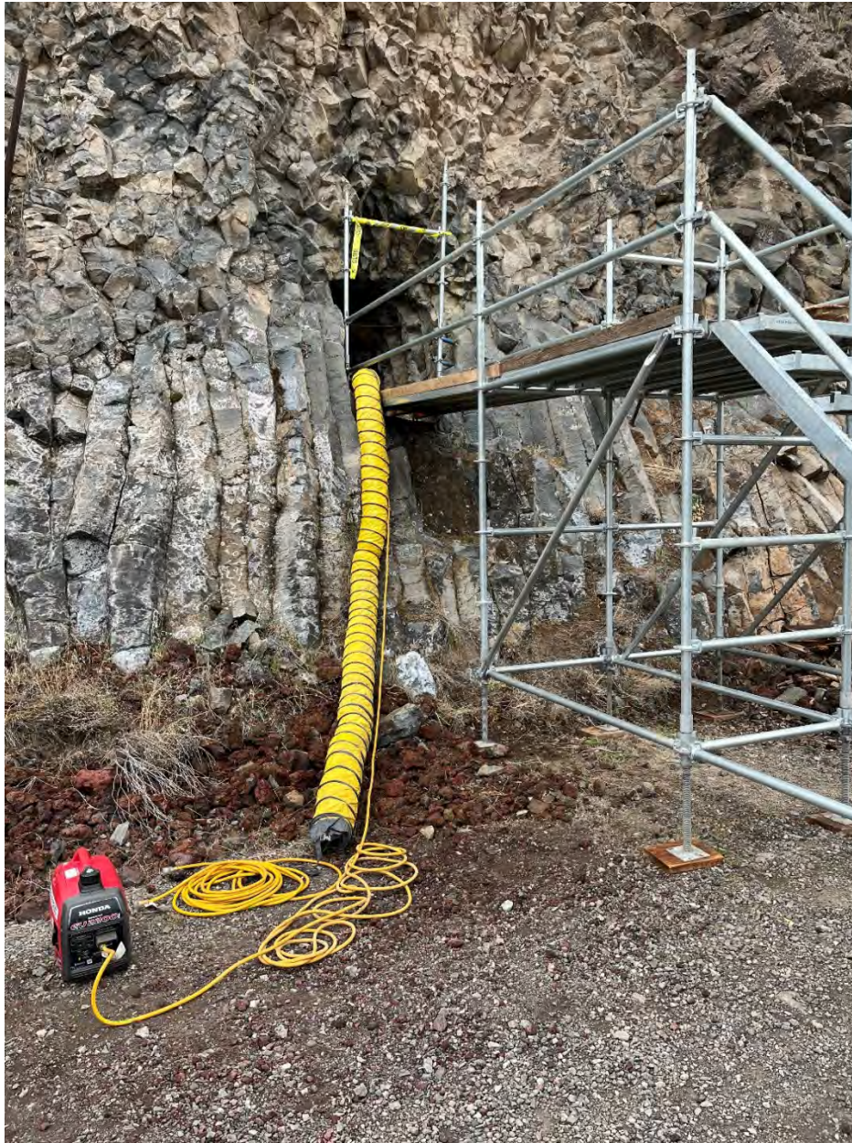
Photograph 1: Cave Venting and Air Monitoring, View 1
