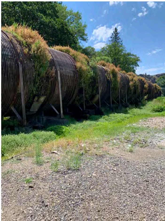
Photograph 3-5: Copco No. 2 Wood-Stave Penstock (Jacobs 2021)
