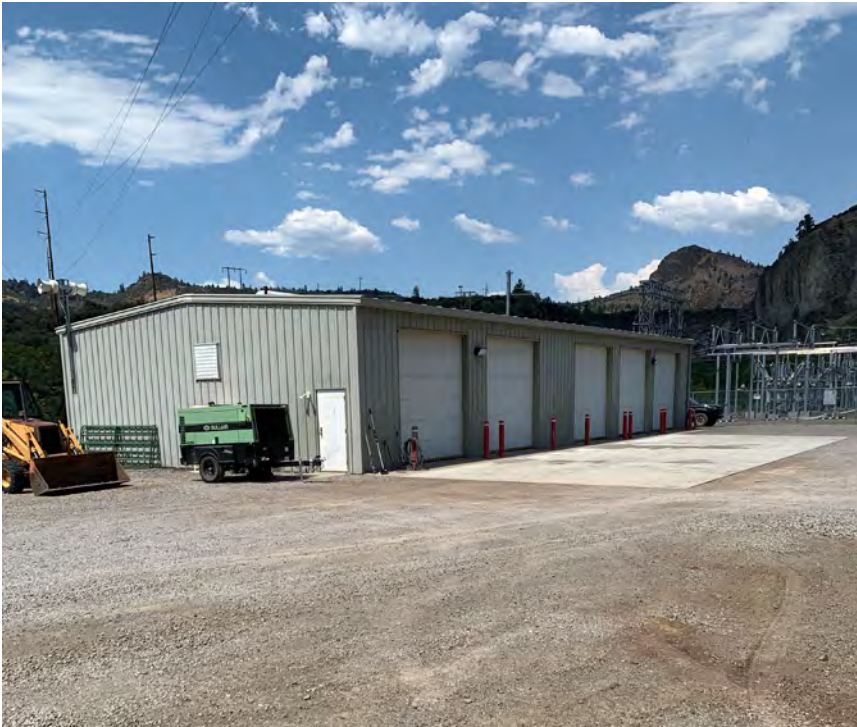
Photograph 3-8: Existing Maintenance Building (Jacobs 2021)
