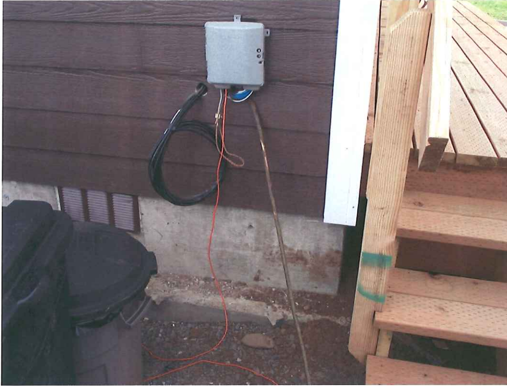
Temporary cable is terminated at subscriber network interface.
