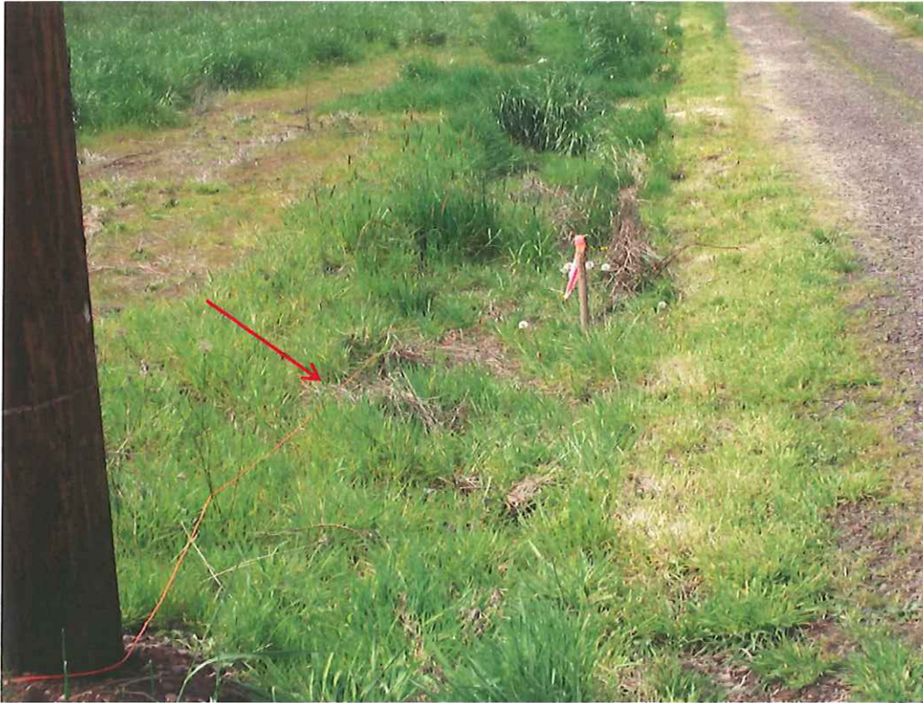
Cable continues west down driveway to 90948 Sunderman Road approximately 200 feet.
