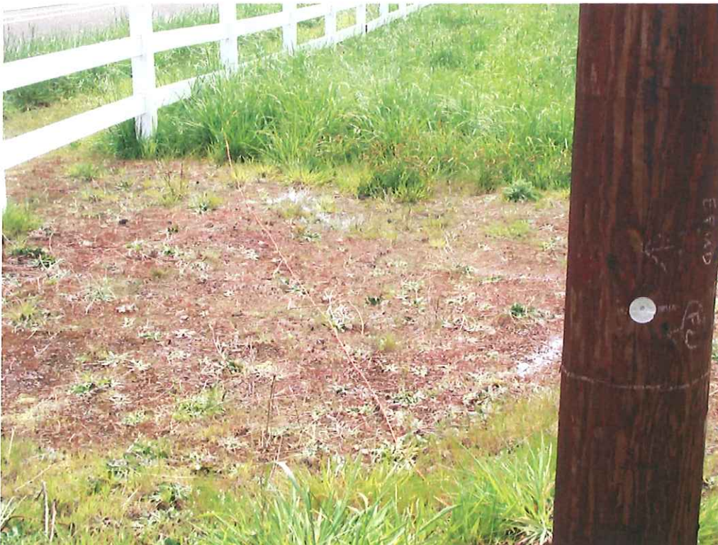
Cable is ground laid north approximately 150 feet, then wrapped around Emerald People's Utility District pole 1602/349604.
