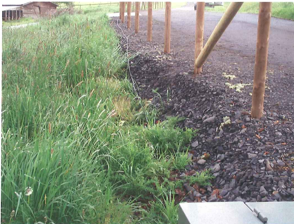
Cable comes out of culvert then continues on south approximately 100 feet.
