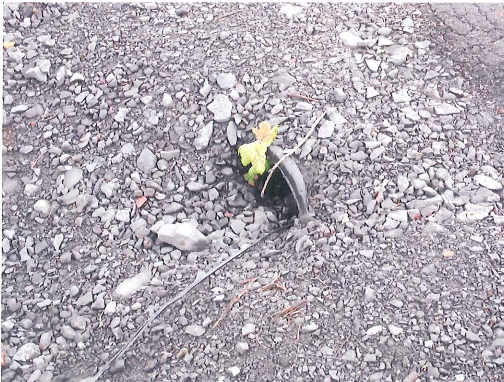
Cable goes under road in culvert then continues on south approximately 100 feet.
