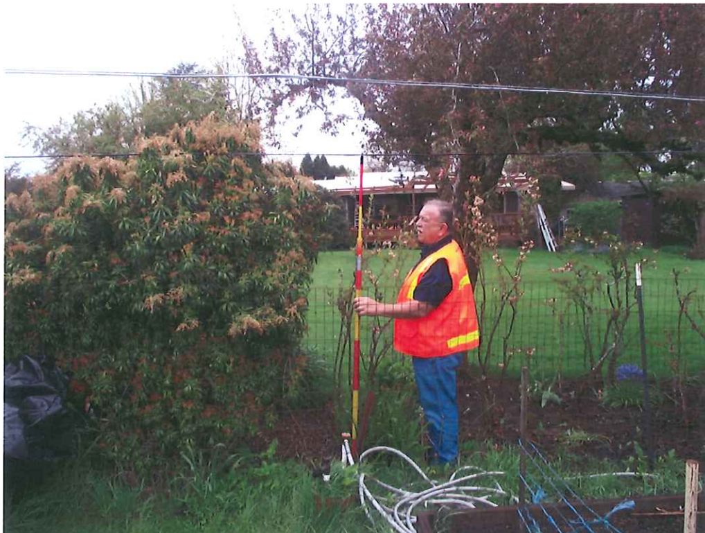
Communication cable has 6'7" clearance above the ground, creating a hazard at 3700 Jackson Street, Corvallis..
