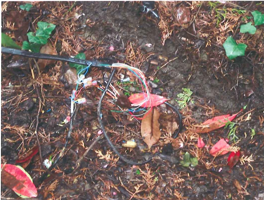
Cable is spliced to a ground laid cable.
