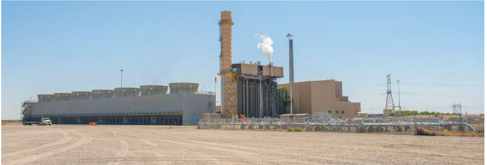
Carty Generating Station, a 440 MW natural gas baseload plant near Boardman, OR
