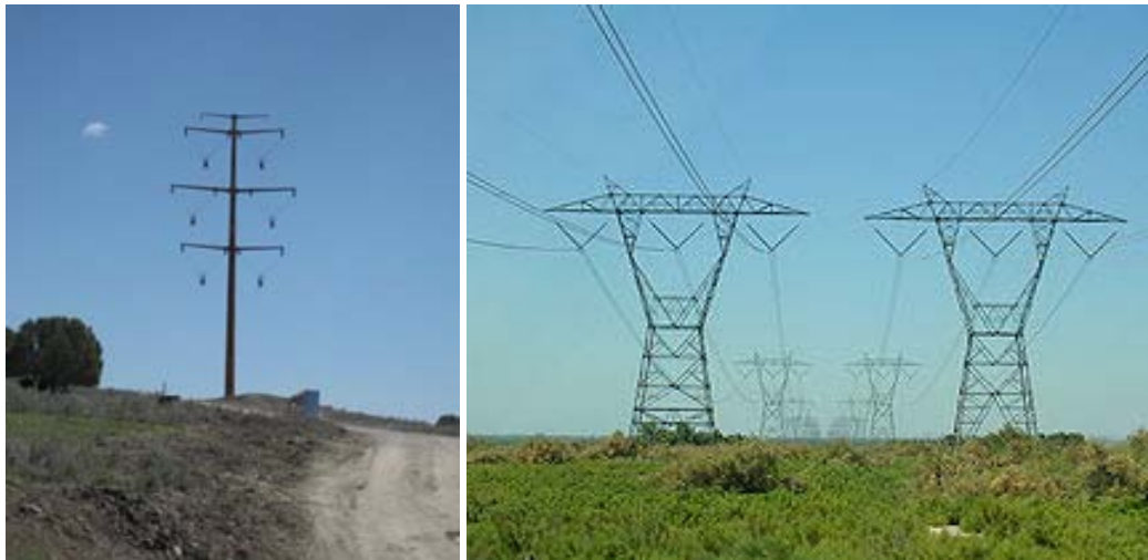
Figure 2-1 Pole Structures: Steel Pole (Populus-Terminal 345 kV) vs. Lattice (Path 26)
