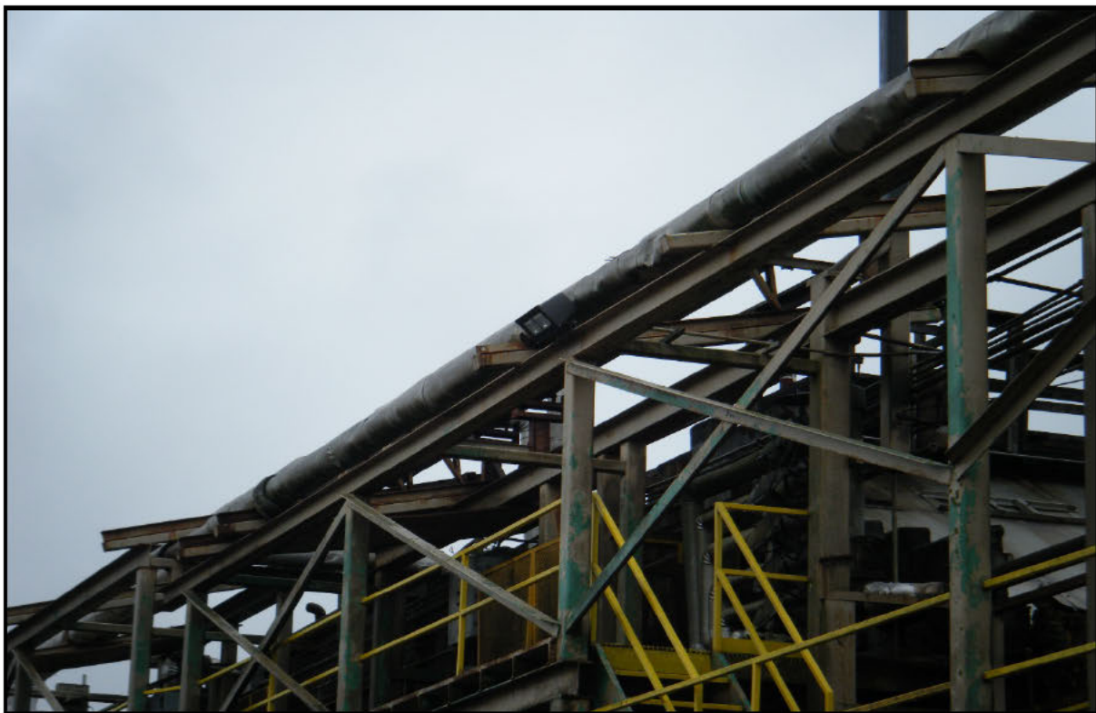
Kiln-12 – Exterior 130 watt LED flood lights installed.
