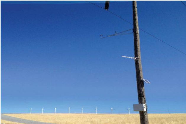
Figure 4. Image of weather station installed near Wind Park
