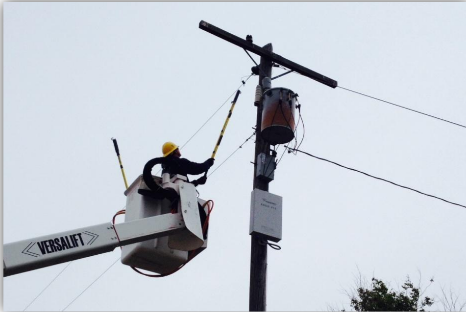
Figure 8. ENGO Unit Being Installed Beneath a Distribution Transformer
