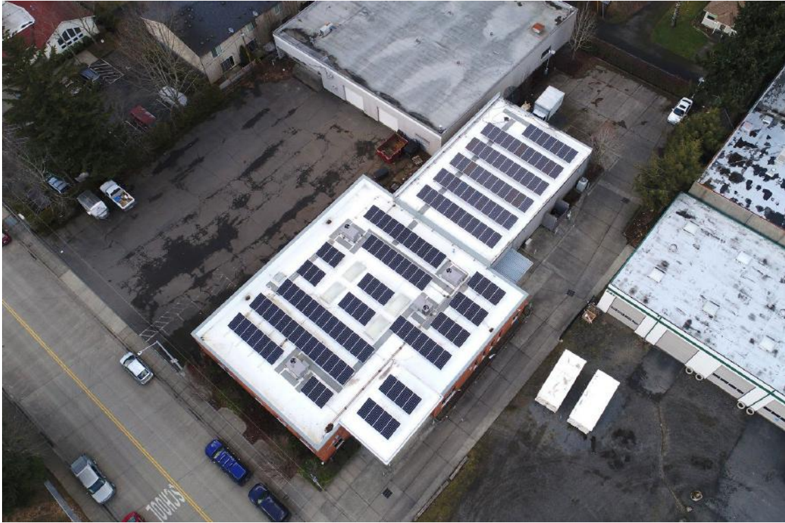
55.2kW Grid-Tied Solar PV System Metroeast Community Media | Gresham, Oregon
