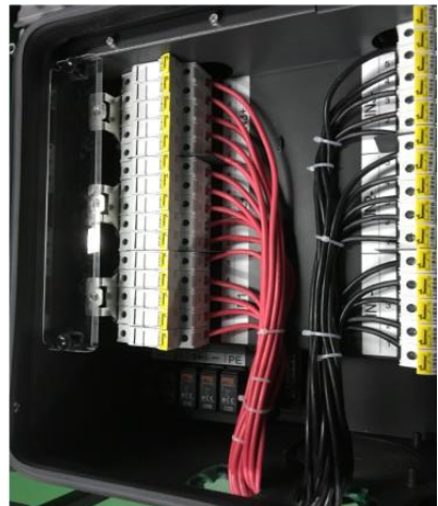
Figure 3-25 DC Input Cable Connection of Standard wirebox
