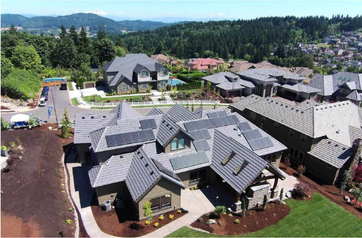
18.7kW Grid-Tied Solar PV System Street of Dreams | Happy Valley, Oregon
