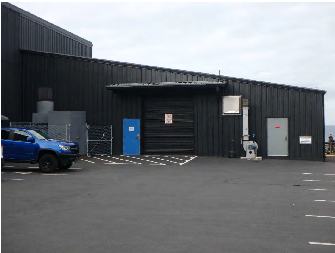
Electrical Room, View from the south
