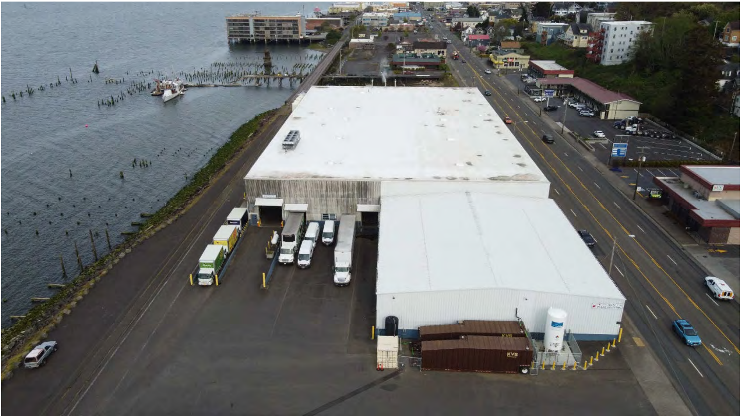
View from the west
