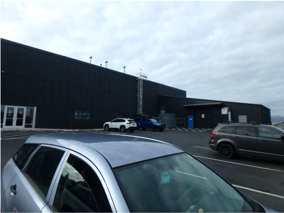
View from the southeast
