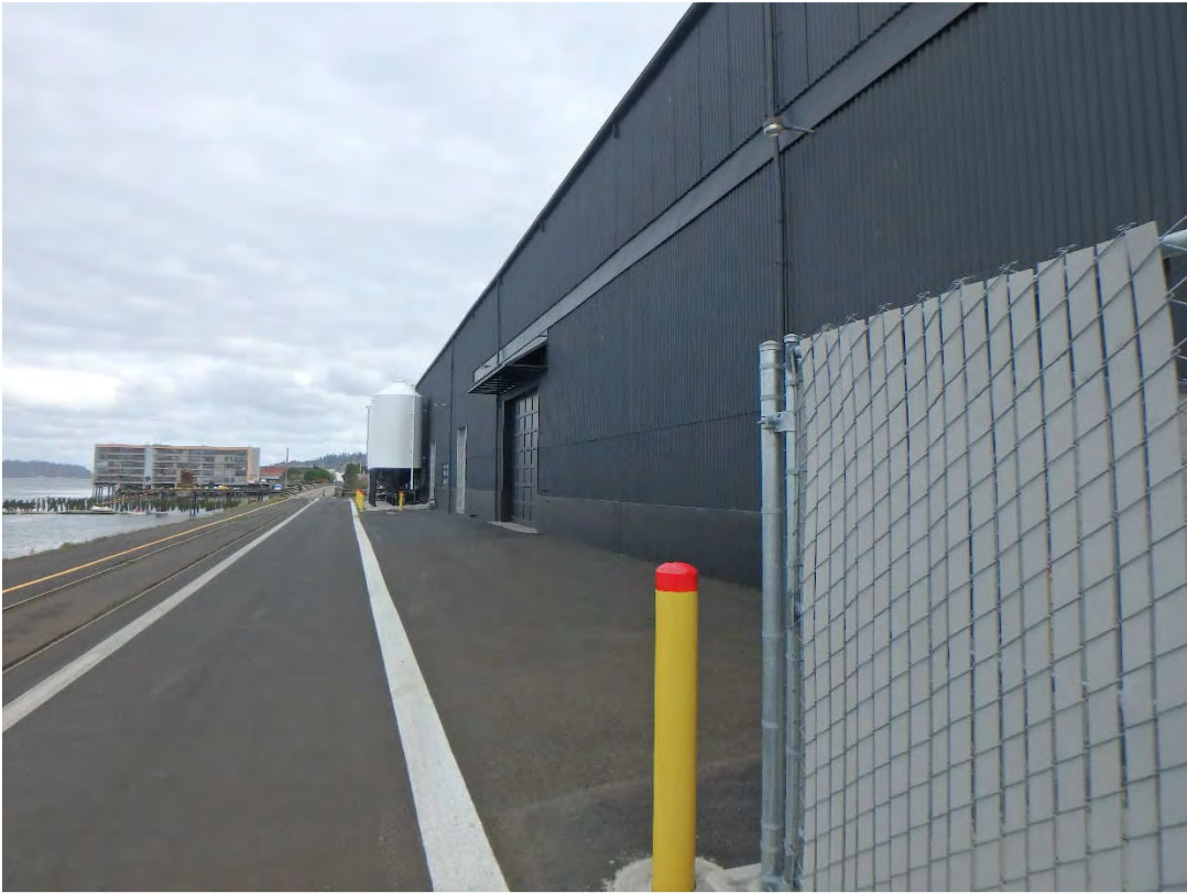
North Side of the building
