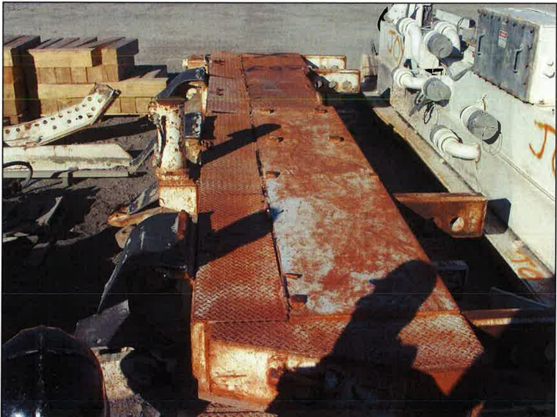
Headgate Drive Platform, 22-214
