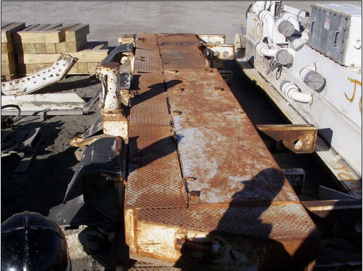
Headgate Drive Platform, 22-214
