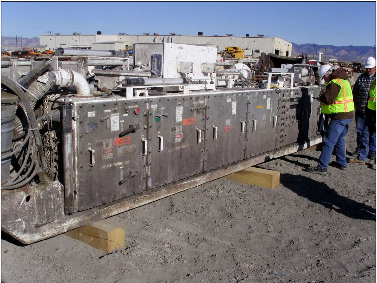
Master Control Station, 22-226
