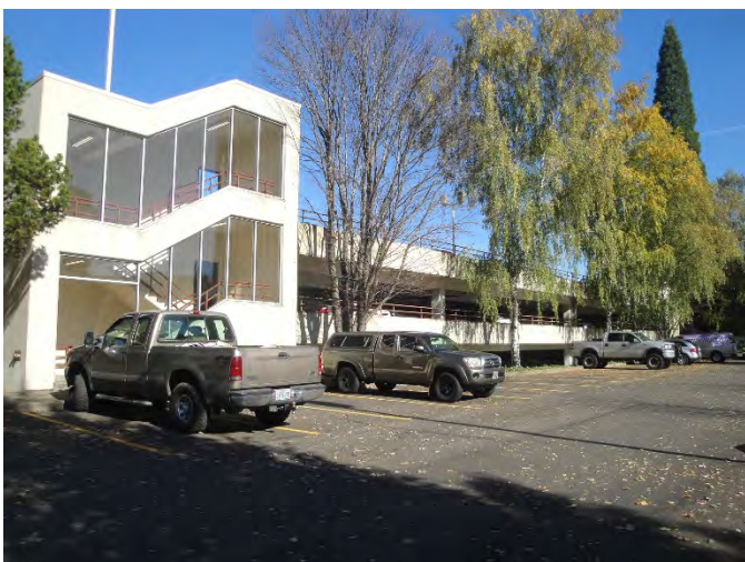
PARKING GARAGE FACING NORTHEAST
