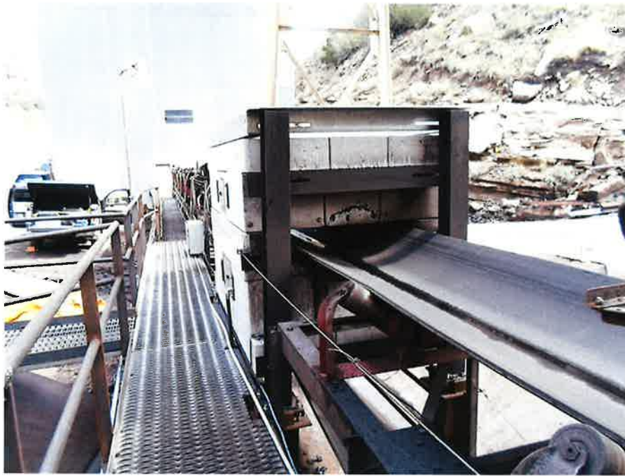
Figure 1.3 ECA Upstream Photo
