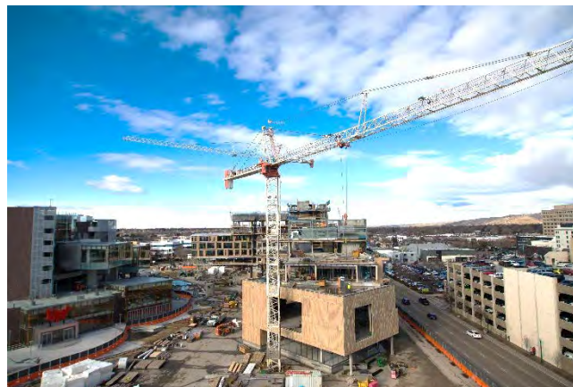
Construction in downtown Boise.
