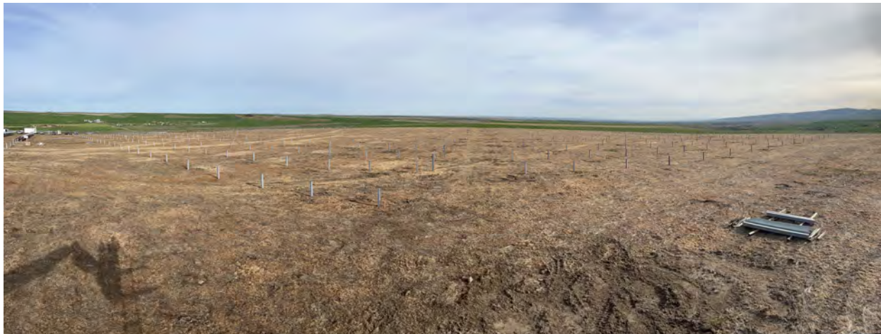
Photo 1. 930 racking & equipment posts installed at Pilot Rock Solar 2 (taken April 11, 2024)
