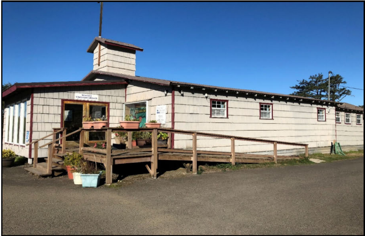
Chapel Hall Exterior – Retrofitted the exterior 75 watt incandescent fixtures to 9 watt LED.
