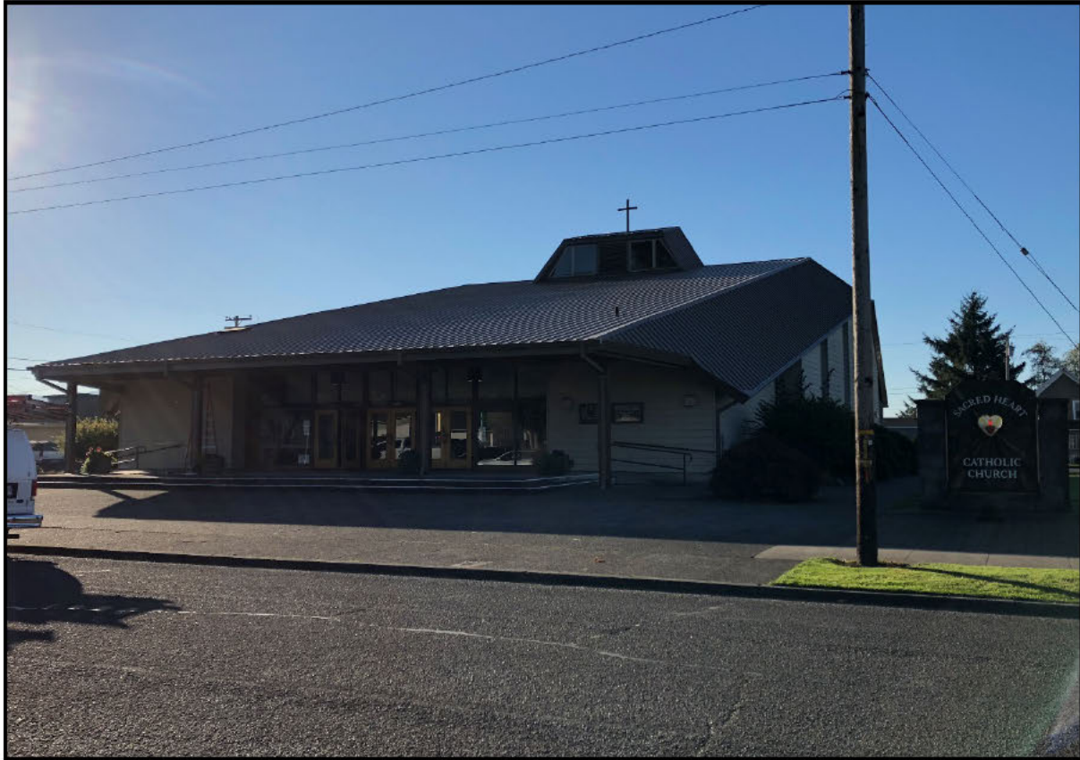
Sacred Heart Parish – Retrofitted the exterior 190 watt fixtures to 28 watt LED.
