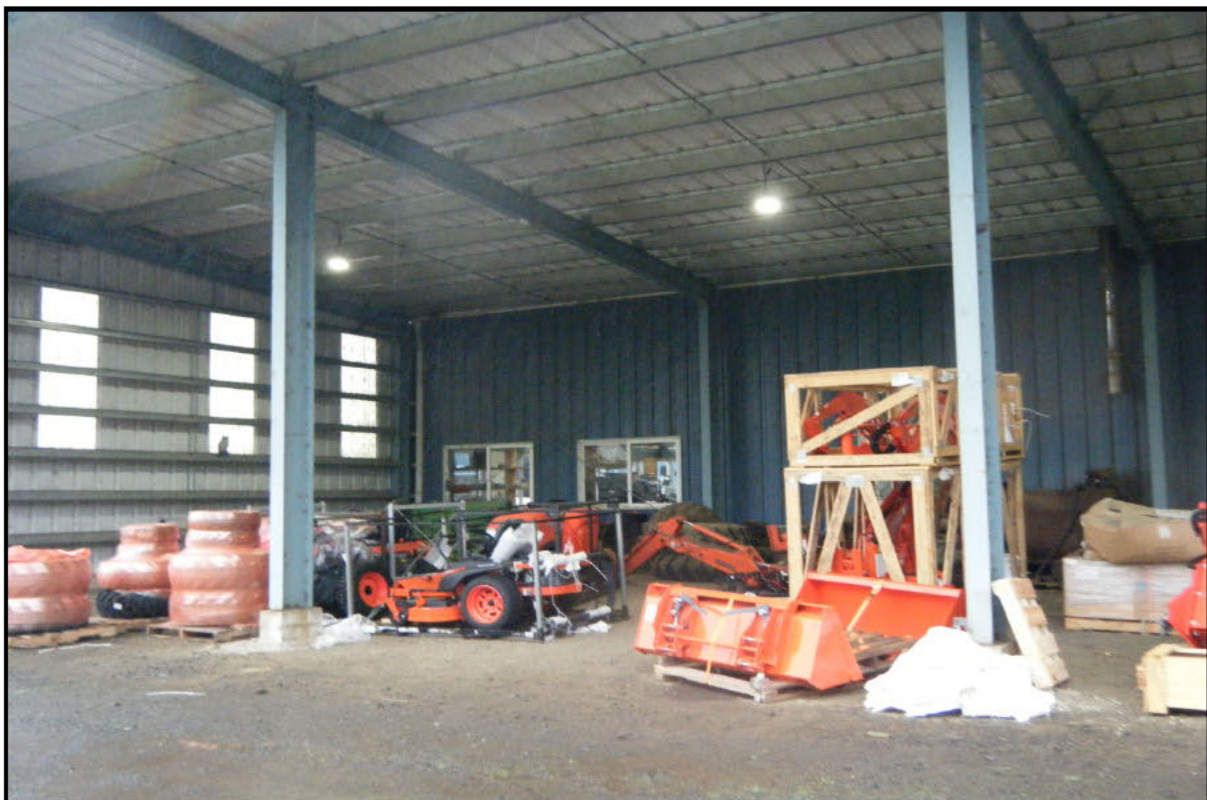
Exterior Lighting – Replaced 500 watt halogen fixtures with 100 watt LED fixtures.
