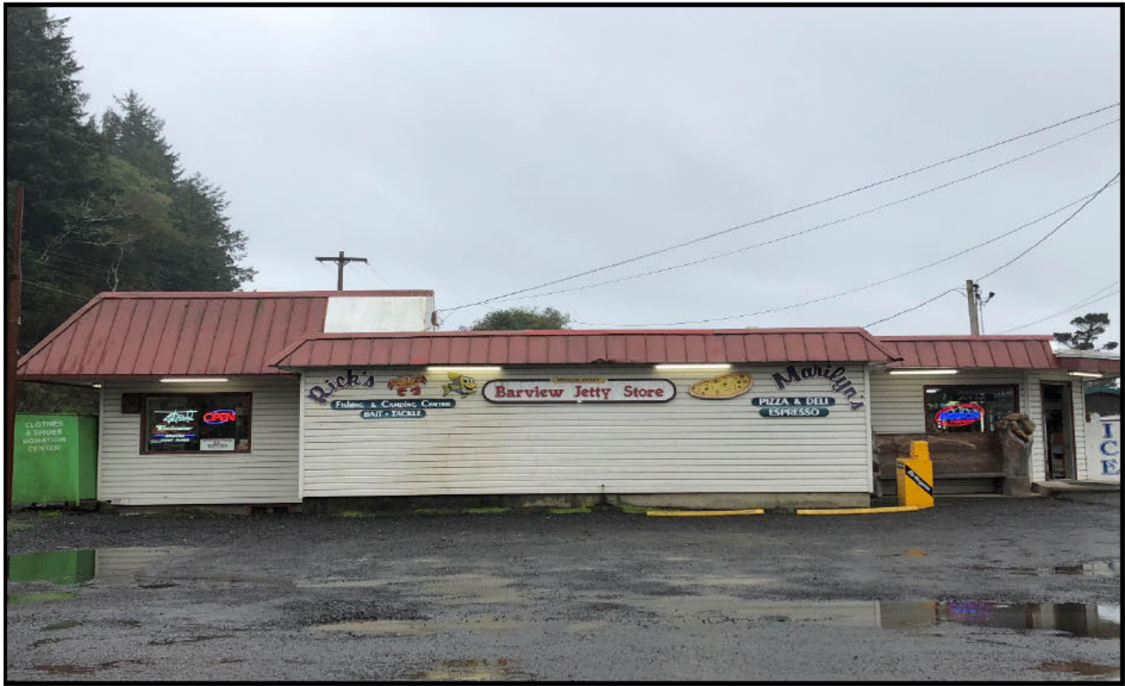
Exterior Lighting - Retrofitted the 93 watt linear fluorescent fixtures to 40 watt LED.
