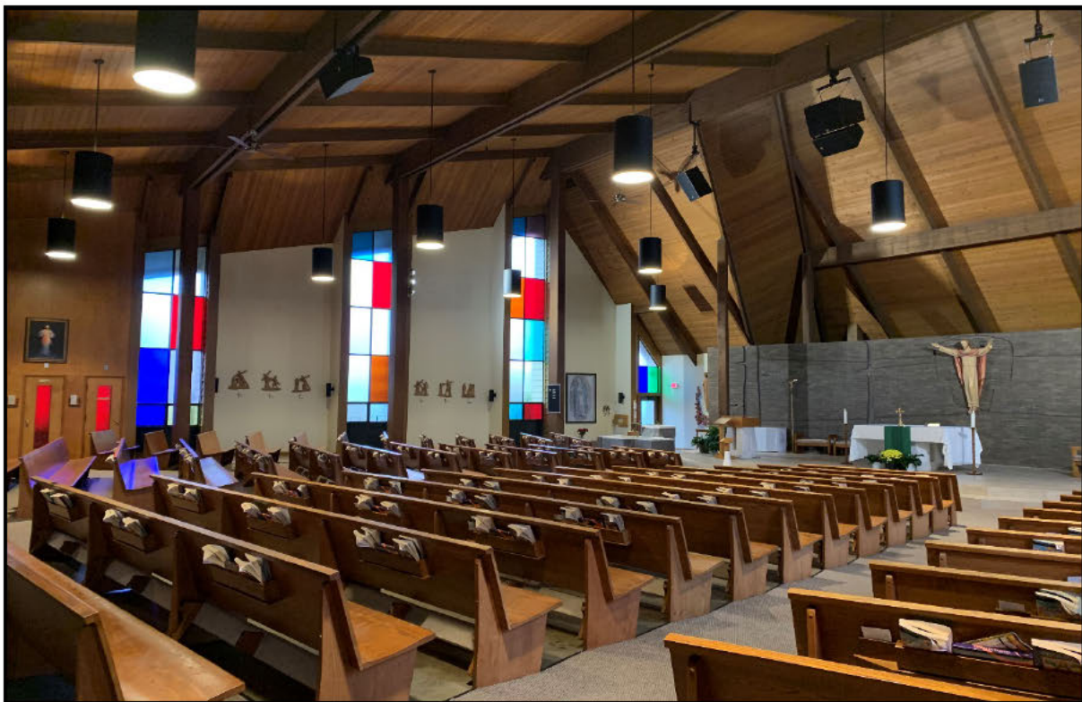
Sanctuary – Retrofitted the 105 watt fixtures to 54 watt LED.
