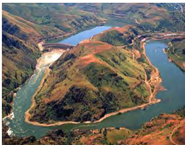
Oxbow Dam, part of the Hells Canyon Complex.
