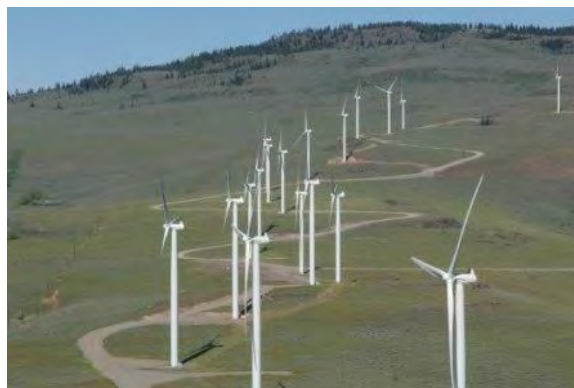
Elkhorn Valley Wind Project, Union County, Oregon
