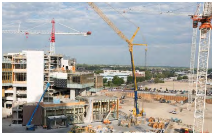
Construction in downtown Boise.
