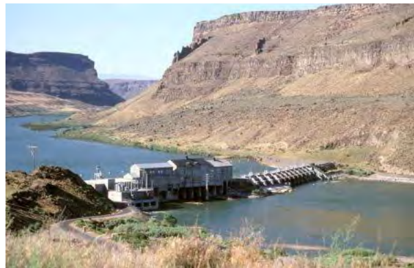
Swan Falls Dam.
