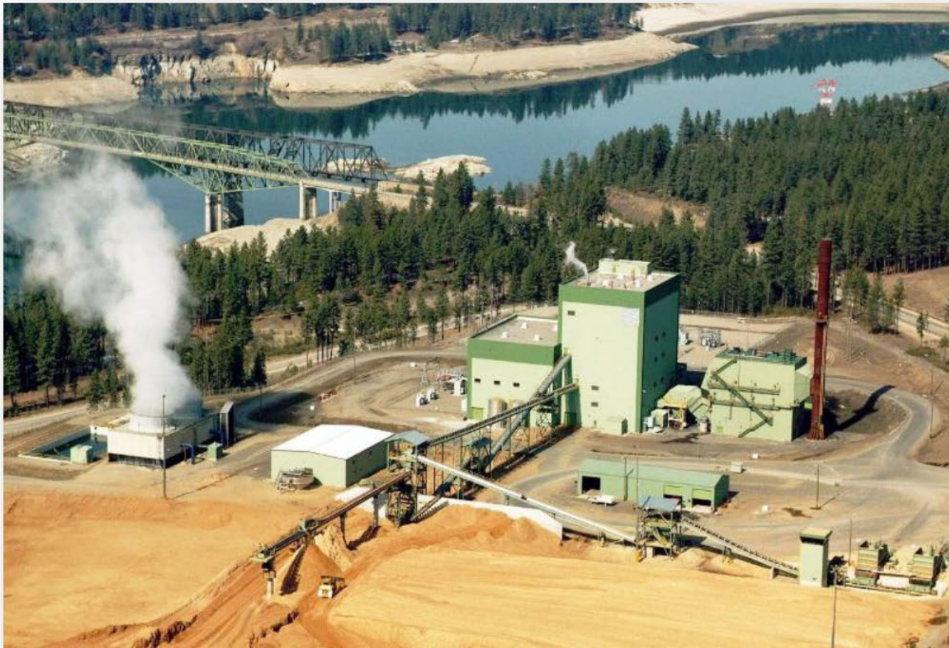
Kettle Falls Generating Station
