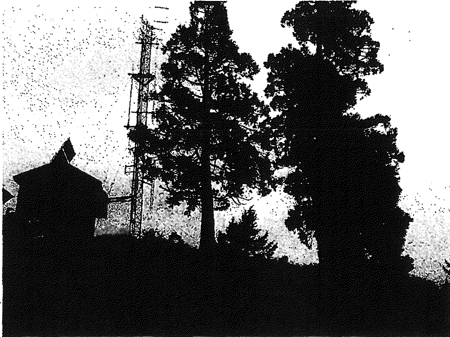
Site Overview. Existing Oregon State Police building and guyed tower.
