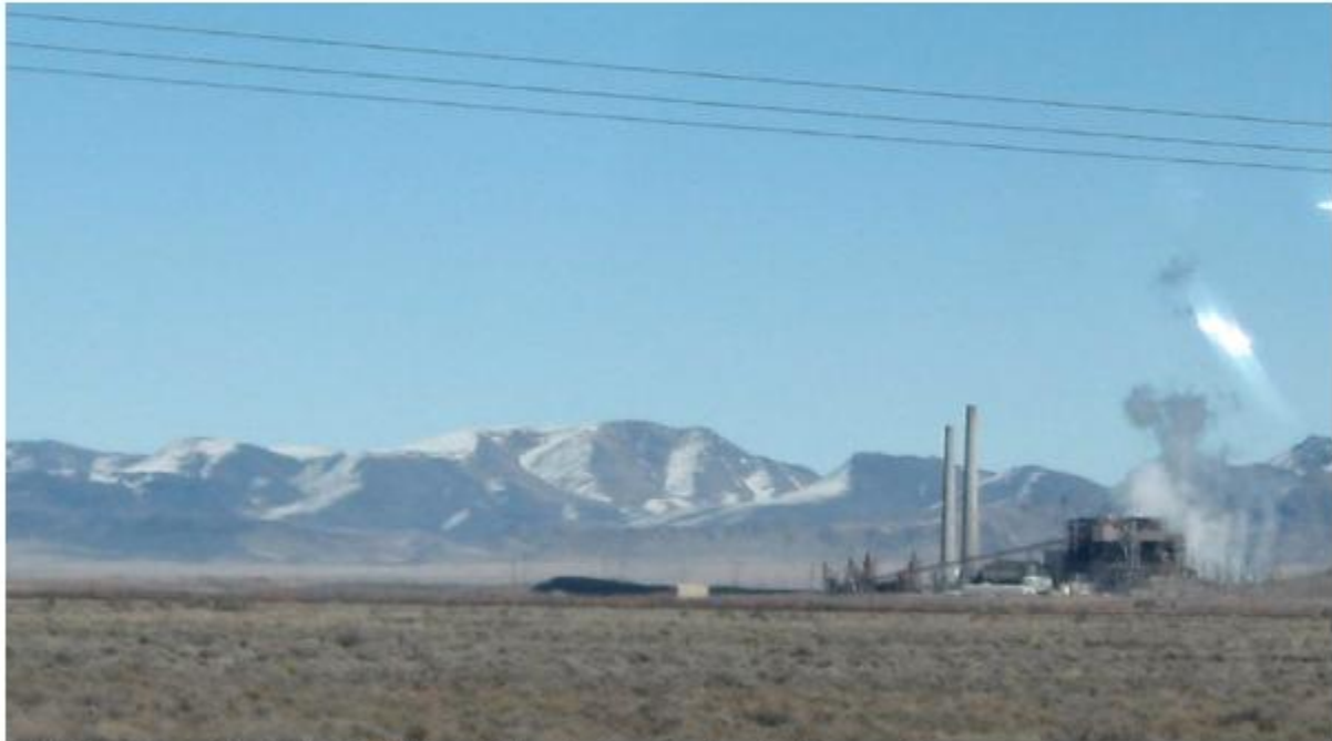
North Valmy Power Plant | Photo: PDTillman/Wikimedia Commons/Creative Commons License
