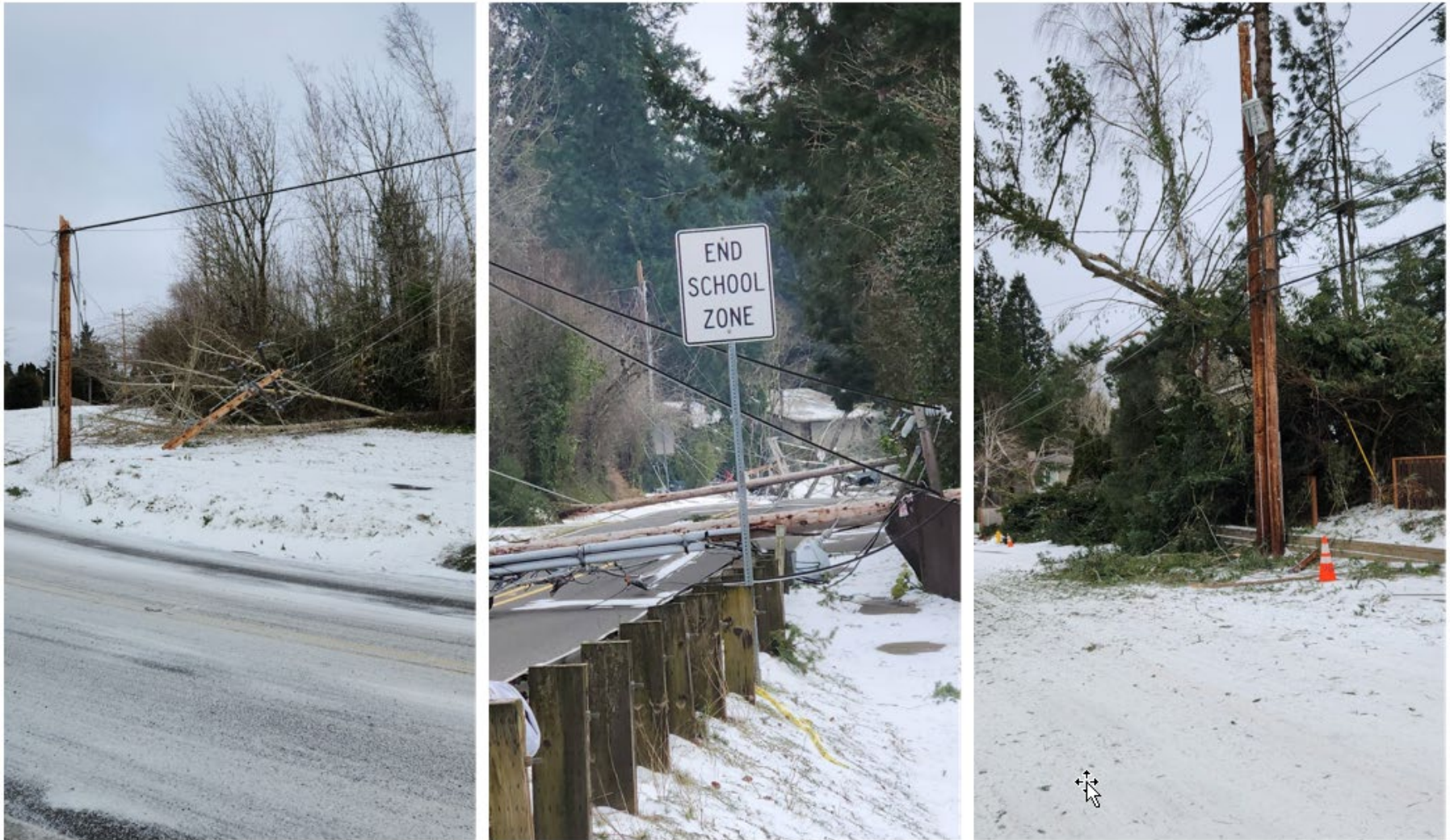
Figure 12: Photos of Extensive Damage and Hazardous Road Conditions
