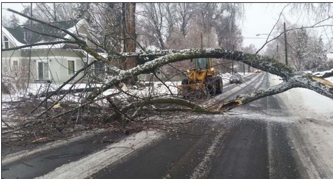
Figure 3 One of several ice-loaded trees which downed lines.
