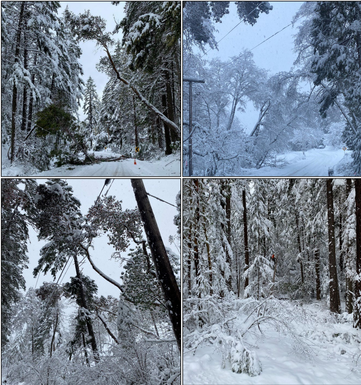
Figure 10: Photos of damages and conditions experienced during the event.
