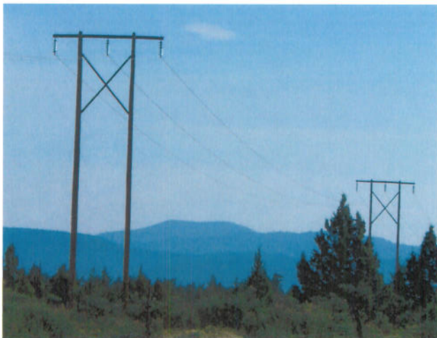
A typical wood pole 230kV structure that may be used in the new transmission line project.
