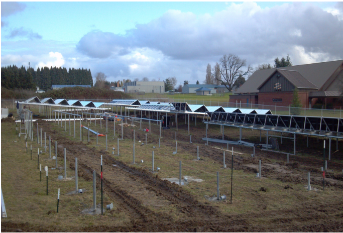
100kw tenk solar system going in at Mt. Angel school
