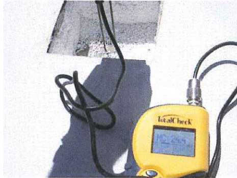
Moisture readings taken at face of lower polyiso layer of insulation.
