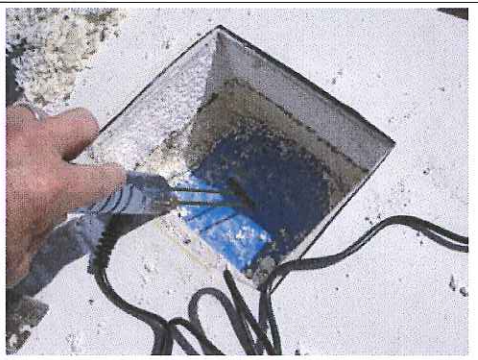
Probes inserted into plywood through cut in vapor barrier.
