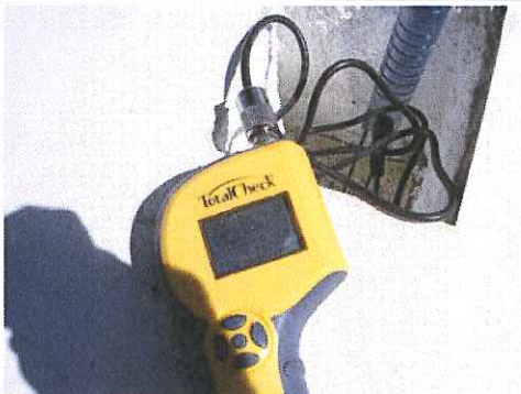
Readings taken through vapor barrier and into plywood sheathing.
