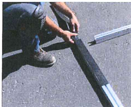
EPDM rubber protection slides easily into rail channel.
