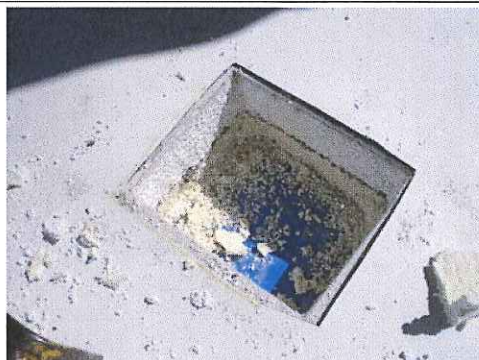
Polyisocyanurate insulation is cut and removed.
