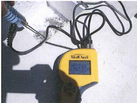
Moisture reading taken at upper portion of polyiso insulation layer.
