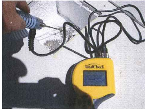
Probes inserted into facer of underlying polyiso insulation.
