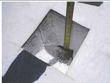
Measurement taken from deck (within insulation joint) to top of assembly.
