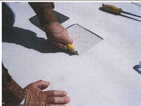
Cover board is cut and removed.
