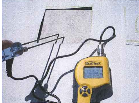
Moisture probes inserted through face of cover board.
