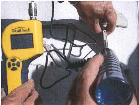
Moisture readings taken within core of cover board.
