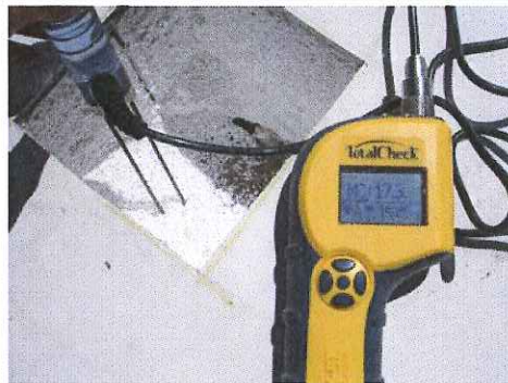
Moisture readings taken at facer of polyiso insulation.
