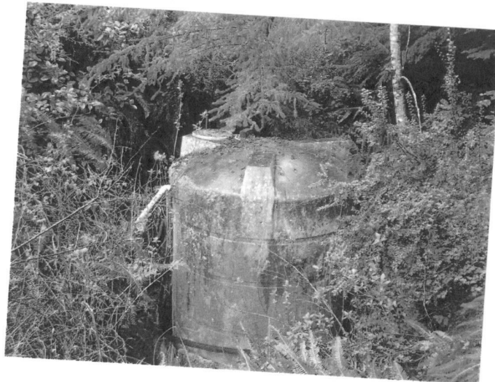
Figure 2-2-1 Existing Storage Tank
