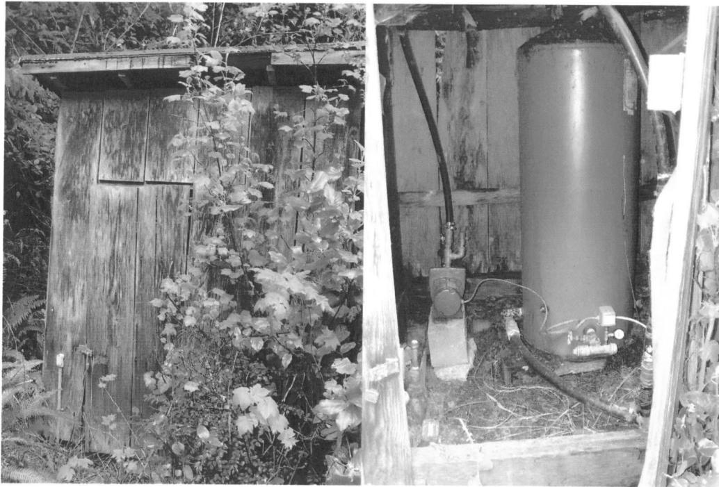
Figure 2-2-4 Existing Pump House
