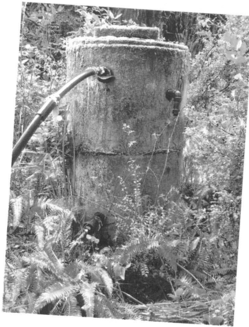
Figure 2-2-3 Existing Spring Box
